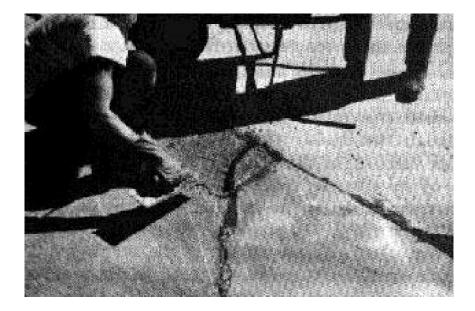
Figure 4 Finishing a patch containing an active crack
